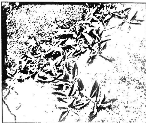
Virginia Buttonweed thriving in a crack
